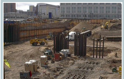
Micropile Deep Foundation
