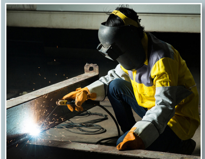
Welding (full penetration welds)
