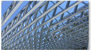
**2211.1.3.2** Trusses spanning 60 feet or greater. The owner or owner's authorized agent shall contract with a registered design professional for the design of the temporary installation restraint/bracing and the permanent individual truss member restraint/bracing for trusses with clear spans 60 feet or greater. Special inspection of trusses over 60 feet in length shall be in accordance with IBC section 1705.2.
