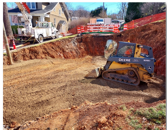
Capping and finishing sinkhole repairs with #21A
