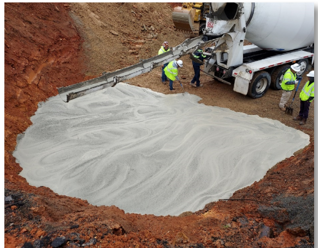
Sealing area with flowable fill near surface elevation
