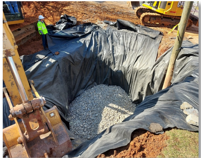
Protecting geofabric with a layer of Erosion Control Stone
