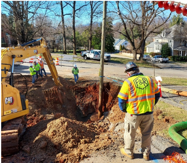
F&R's Hoyt Alford observes the excavation of a sinkhole
