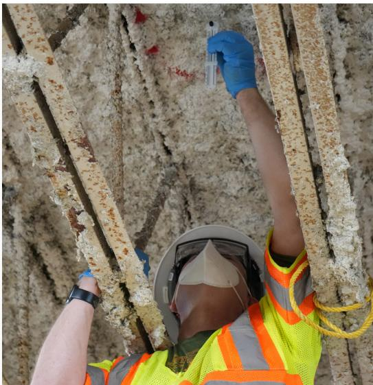
not limited to, substrate temperatures and surface conditions; SFRM handling, storage, mixing, and conveyance; method of application; curing; and ventilation. (Note that in this specific case, the IBC code adopts the manufacturer's recommendations and makes them code law.)
