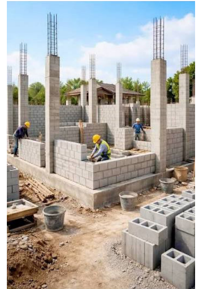
Masonry Construction with CMU
