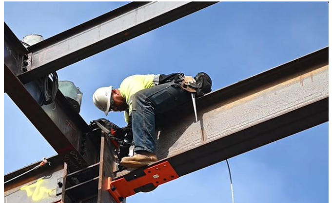
Structural Steel Inspection – Bolted Connections (Image: BE Blog - Simpson Strong-Tie)
